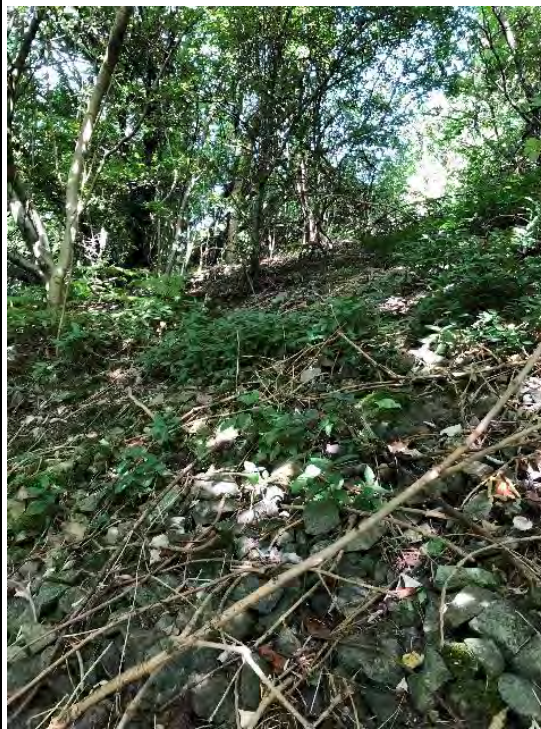
Photograph 42: IMG_3358. Photograph of counterfort drain in hillside. Drain is gravel filled and approximately 3.5 to 4m wide. Photo looking 350°.
