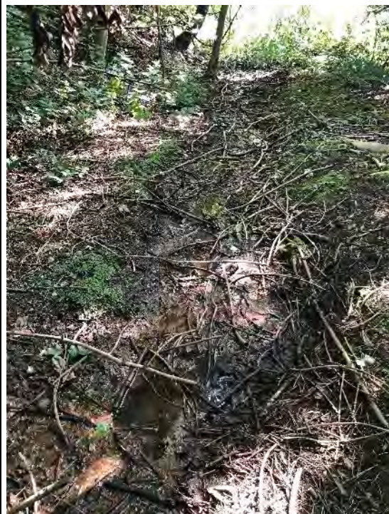
Photograph 38: IMG_3358. Photograph of spring emerging from drainpipe in rock slope. Rock slope is likely to have been benched but look fairly irregular. Photo looking 120°.
