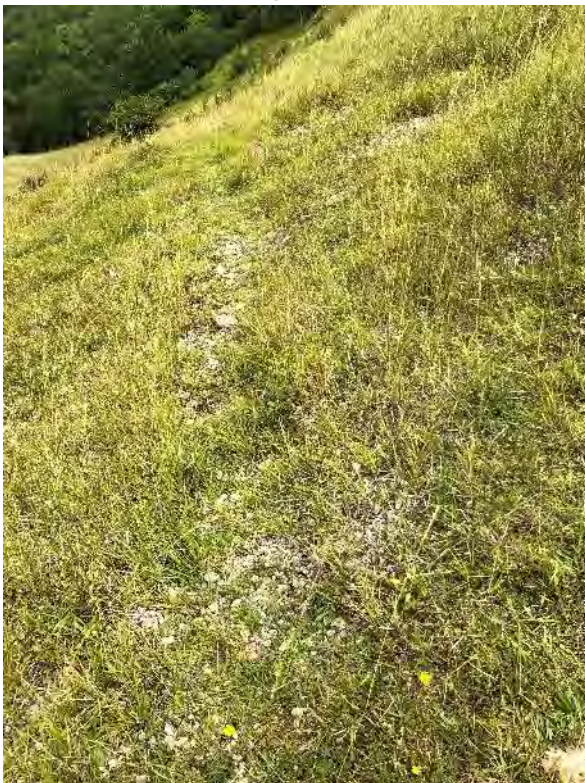
Photograph 9: IMG_3248. Photograph of scree slope in line with source of boulder, coarse gravel sized limestone (IO) fragments up to 500mm long cobbles. Photo looking 020°.
